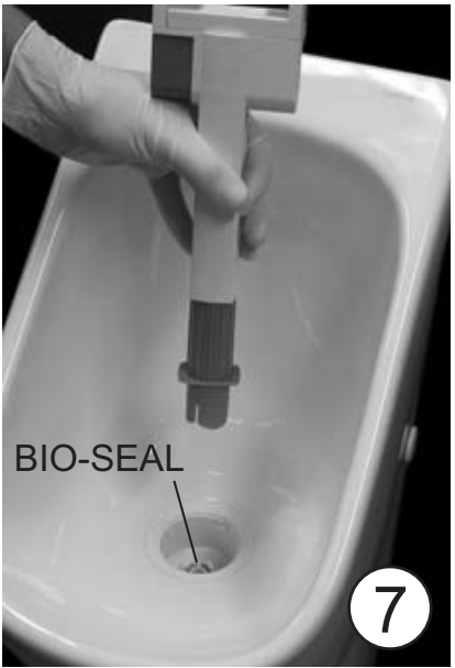
INSERT TOOL CAP AND LOCATE ON BIO-SEAL
