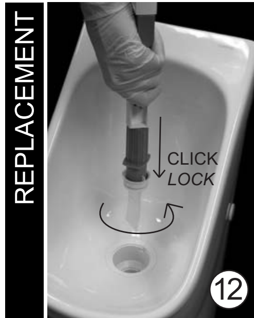
INSERT NEW BIO-VALVE AND ROTATE ANTI-CLOCKWISE TO LOCK
