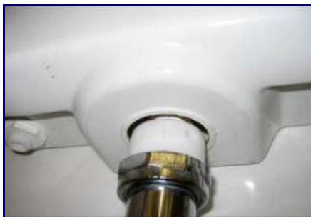
Align & connect Physical Air Gap
