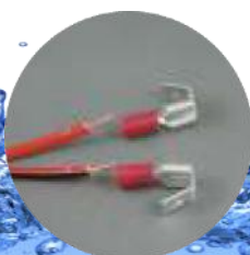
Place the Piggyback connectors and crimp them to the wire.
