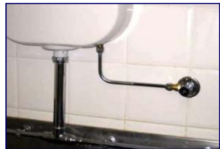
Connect all thread tubing to inlet pipe via stop tap
