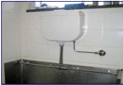
Typical Concorde Urinal Cistern
