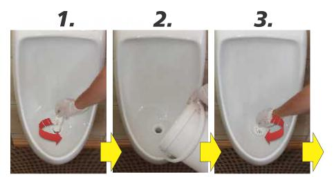
Remove D-Valve with Service Key counter clockwise and dispose
