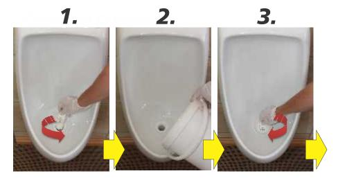
Remove D-Valve with Service Key counter clockwise and dispose
