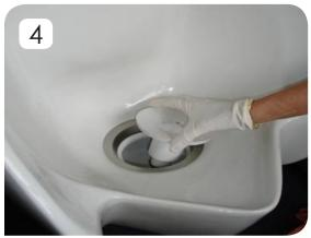
Take a new Drain Insert and place it in the waste trap.
