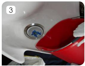
Rinse the trap with two buckets of warm water. If necessary, use a small brush around the stainless steel ring. **Be careful not to scratch the ring.**
