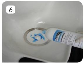
Pour about **30 oz. of water** over the Drain Insert. Then slowly pour the **entire contents of the Odor Barrier** onto the Drain Insert. Wipe clean. The ZeroFlush<sup>®</sup> Urinal is now ready for use.
