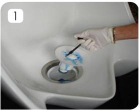
Screw the key into one of the holes of the Drain Insert and pull upward to remove. When insert is pulled, the contents of the waste trap empties into the waste line.
